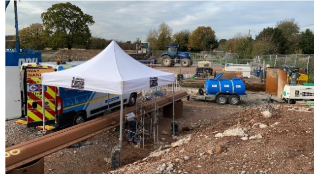
Figure 6. Bi-directional loading test underway (Fugro).
