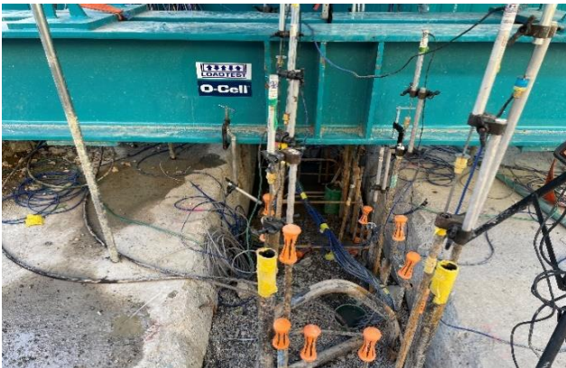
Figure 2. Bi-directional loading test on a pile with concrete cut-off level 12.3 m below ground level (Fugro).
